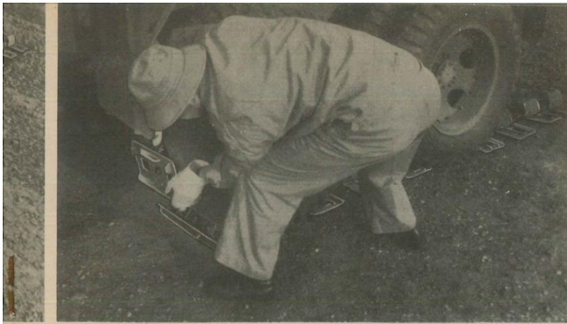
Figure 5. Joe tilts up the first few track shoes and holds them firm against the tire. When he's all set—feet away from the track—he yells, "Gung ho!" and the driver backs up some more . . . slow.
